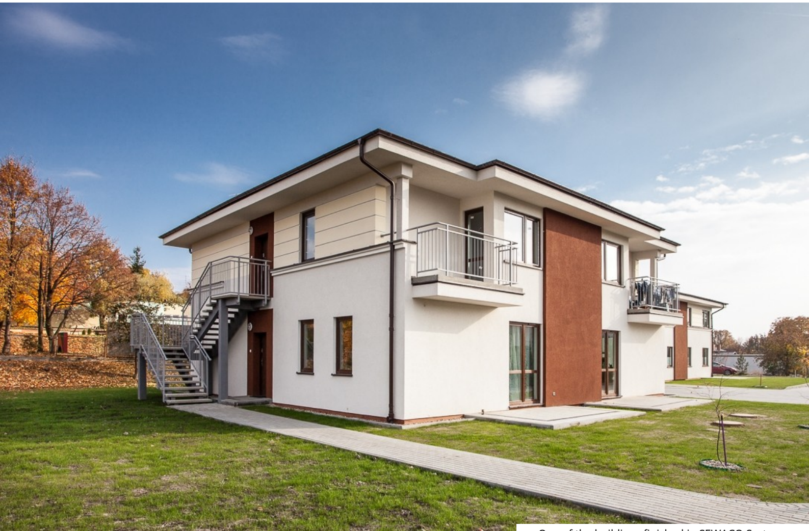
One of the buildings finished in SEWACO System
