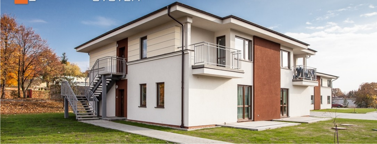
One of the buildings finished in SEWACO System in 2013
